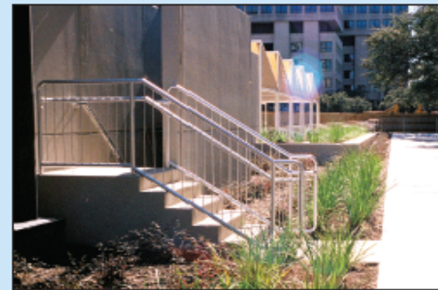
Figure 3-25. Three sets of stairs that provide building egress during the design flood event, but still allow normal use of the building (source: Walter P. Moore)
